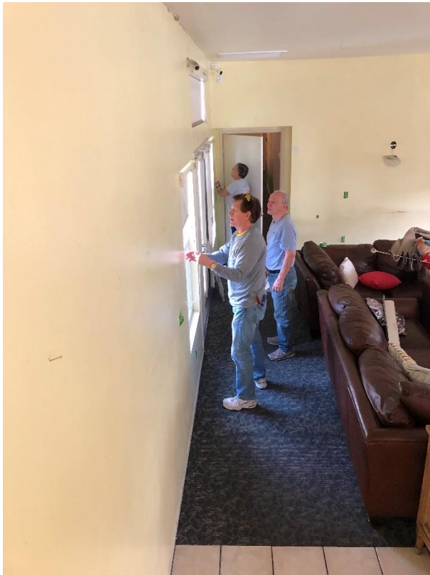
Mike Cushing, Tony Giusiana, and Roy Alcocer inspecting the yellow wall.
