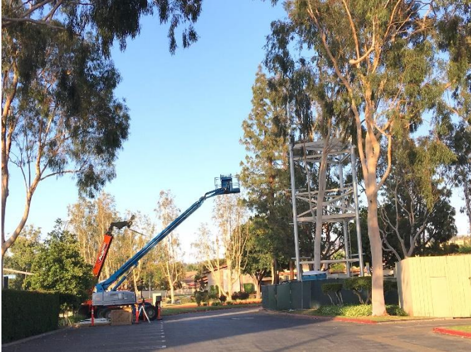
Progress is being made on the cell tower to the right.
